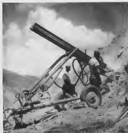
One hundred and fifteen units of mechanical equipment have been used in the highway construction. This view shows the drilling equipment used to make holes for dynamiting rock sections.
